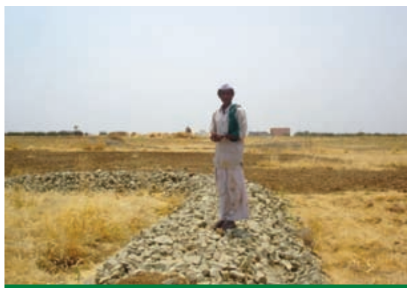
A farmer atop a loose boulder structure constructed on his field
