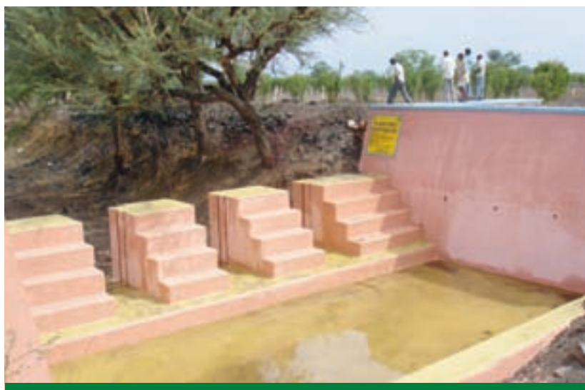
A masonry stop dam constructed under the Sunhera Kal project
