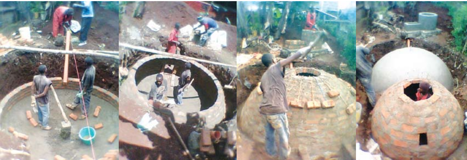
Construction of Biogas plant in progress, Caimbaba village, Kakyu district, Kenya
