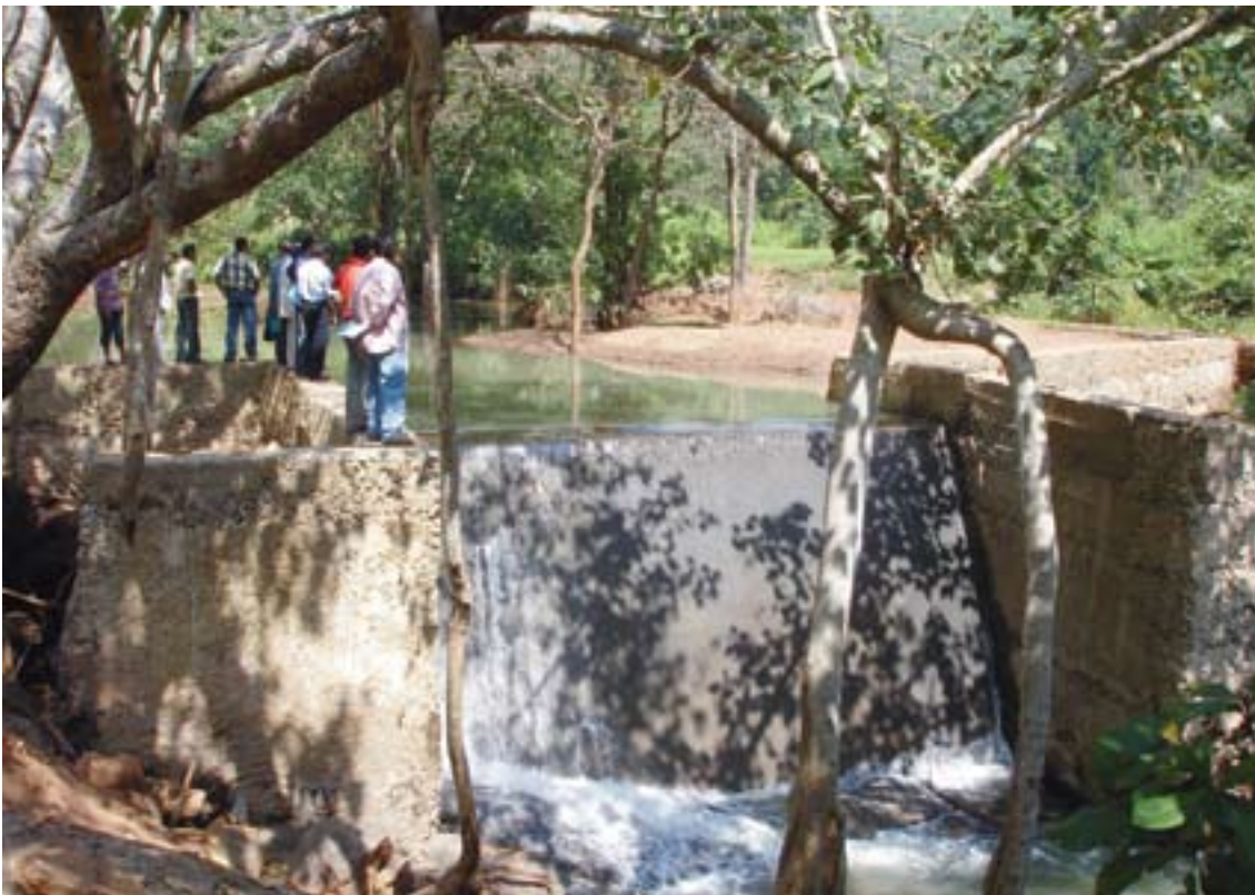
The check dam constructed in the Burdakia Nallah watershed
