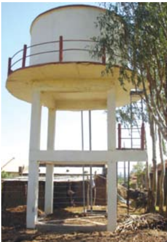
An Elevated Storage Reservoir (ESR) constructed at Village Kasarshirambe
