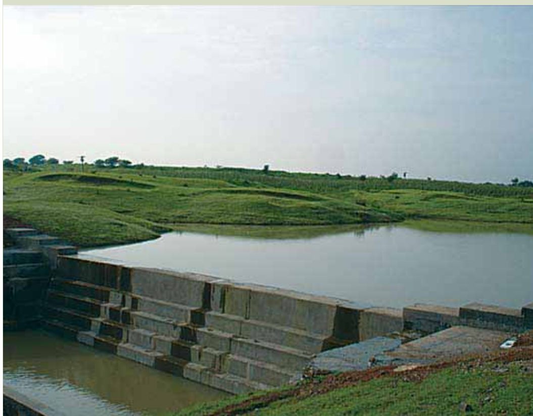
Masonry stop dam constructed in village Chhatargarh World Vision India, ADP- Ratlam
