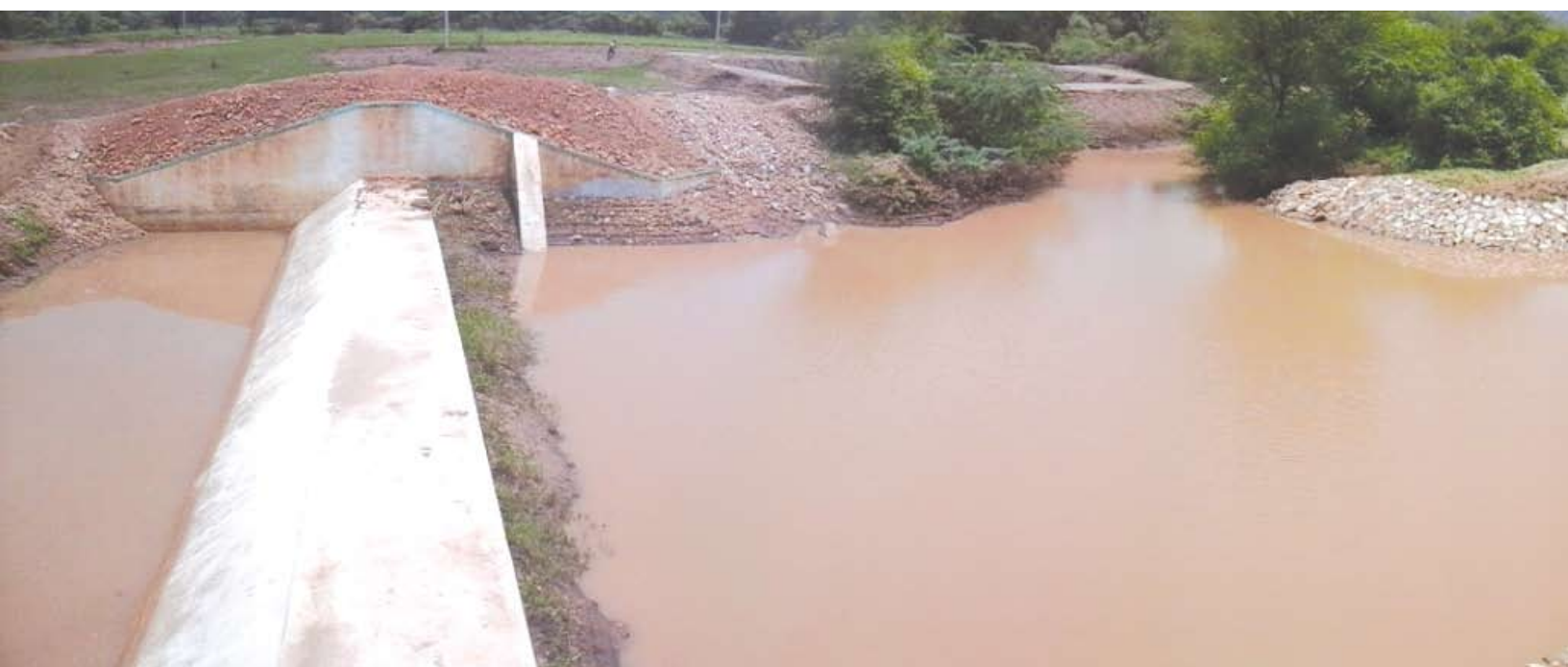
Construction of anicut
