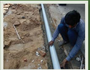
Connecting the underground pipe to the collection pit
