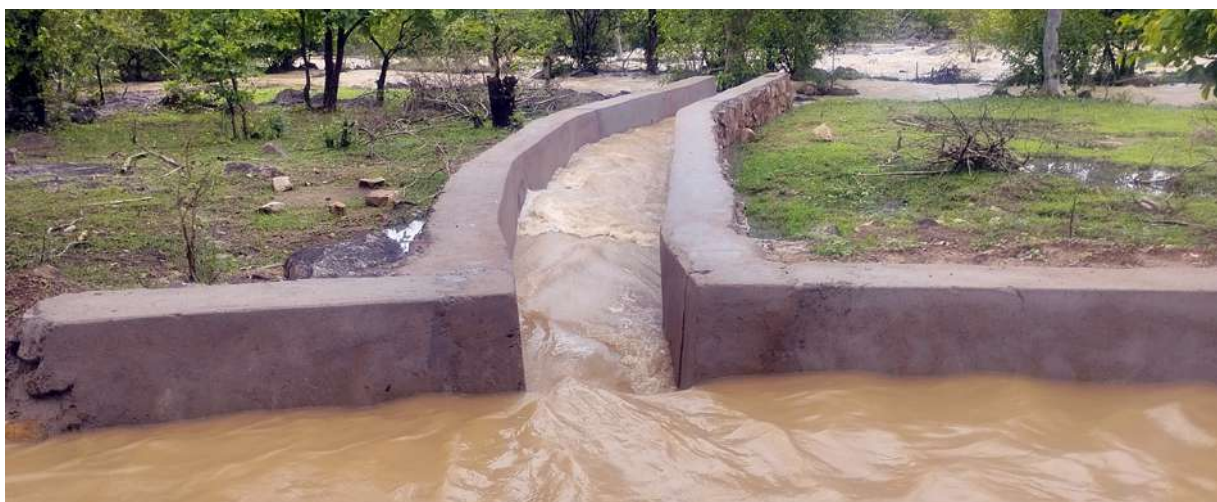
Lined Nali construction for irrigation support to farmers in Hitiksha Village, Chhattisgarh
